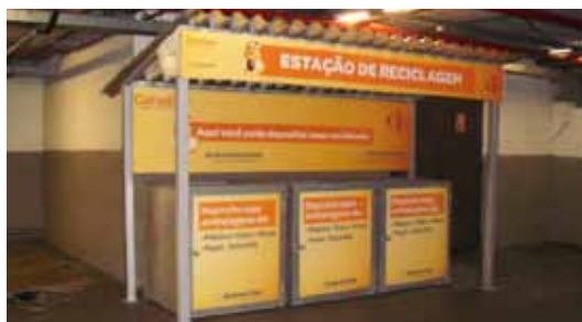
The recycled garbage collecting stations of 10 Carrefour stores were built with recycled plastic sheets.
